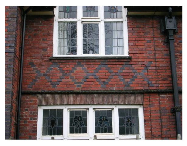
FIGURE 9: Diaper brickwork and tile window heads.
