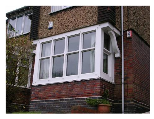
FIGURE 10: 13 Victoria Park Road – wet dash render above smooth red brickwork
