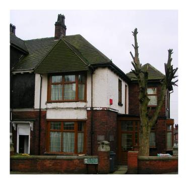
**FIGURE 19:** Harmful modifications. Removal of timber sash windows and replacement with inappropriate uPVC.
