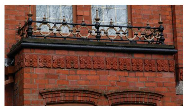
FIGURE 7: Façade finishes: Flemish bond brickwork with moulded brickwork frieze panels.
