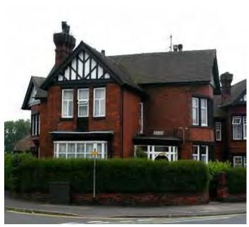
sides with 2 horizontal projecting courses near top of stack. Stepped brickwork under cap. Pilasters widen and run up cap, 3 pots. No. 2 – as for No. 1 chimney from projecting course upwards.
