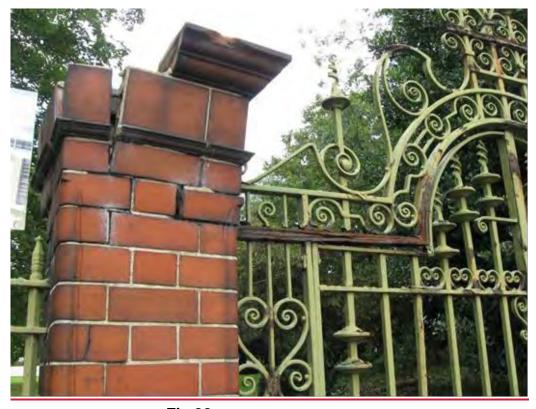
Fig 38: Gatepost in poor condition
